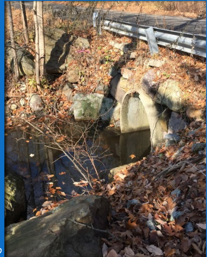
Valley Road Bridge, Rockaway Township
